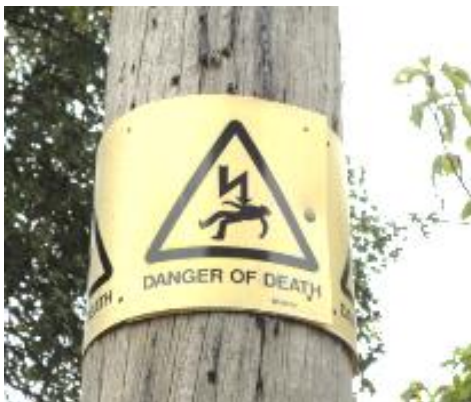
Example of LOW voltage joint user pole sign "DANGER OF DEATH"
