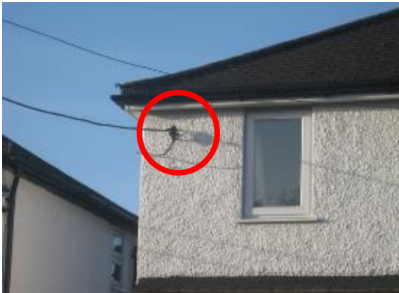
Example of a concentric neutral service (a single cable) separation at attachment of 200mm.
