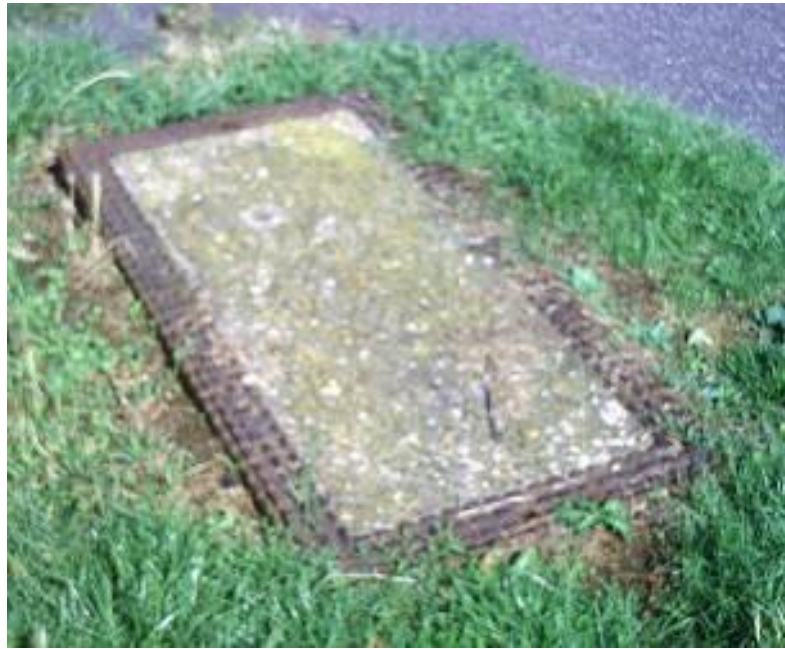
Figure 13: Castellated cast iron cover
