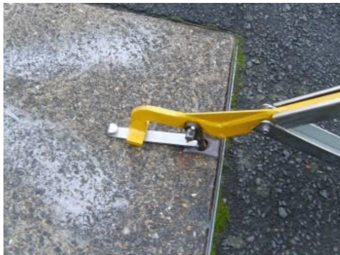
Figure 16: KJB No.5 and KISS tool prior to removal of chamber cover.
