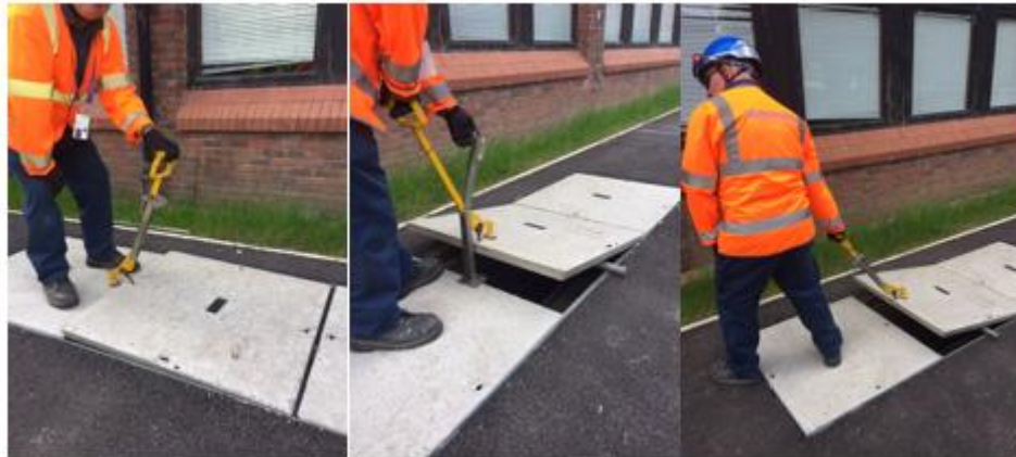
Figure 8 - JF 10 &amp; 11 Cover Removal
