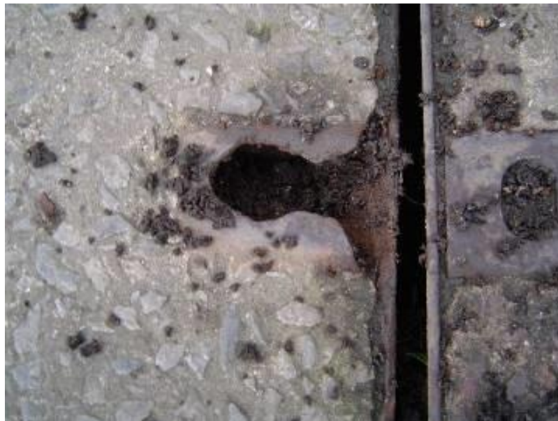
Figure 12: A corroded keyhole
