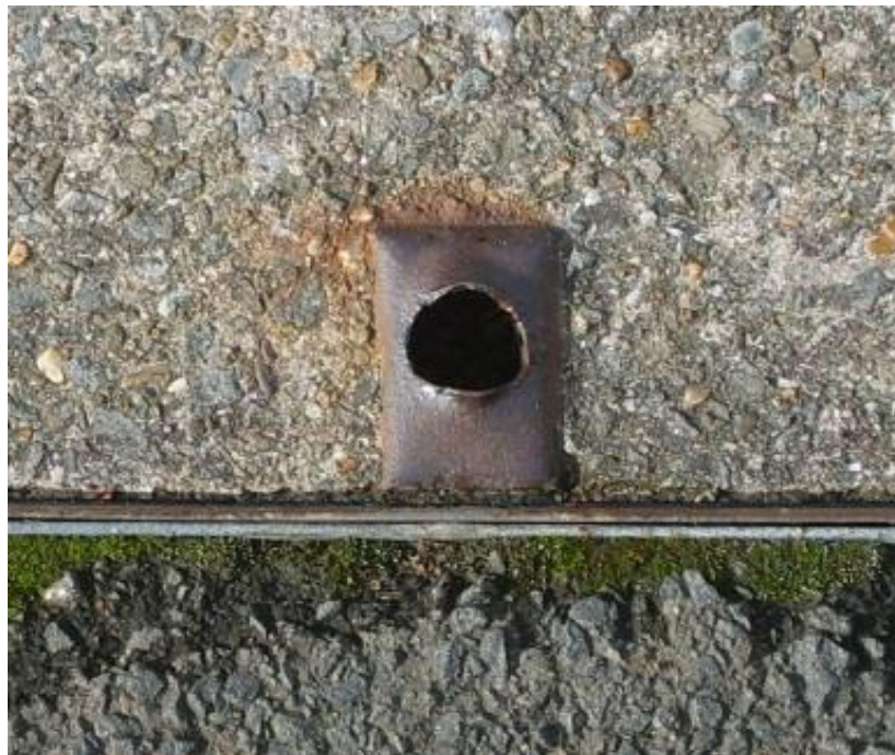
Figure 11: Above: A typical worn chamber cover keyhole
