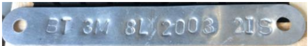
Figure 6- Aluminium strip close up, showing owner (BT), 3 Metre mark (3M), pole size and class (8L), year of preservation (2003), supplier (2) and finally the Depot (IS)
