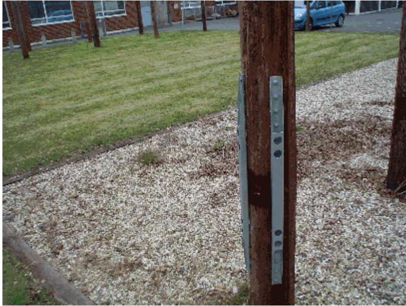
Figure 37: Completed repair – metal straps fitted
