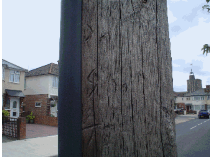
Figure 3- Although still just visible, the 3m mark is becoming faded
