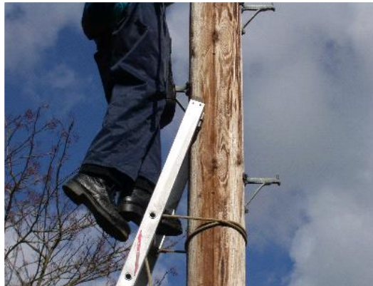
Figure 31: Shows the ladder position, with the right leg about to swing round to the first step
