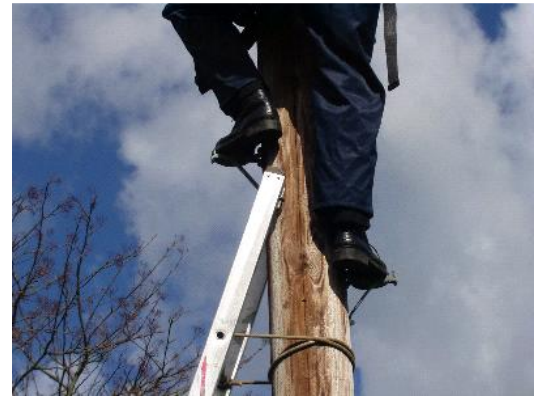
Figure 32: - shows the right foot in position and the climb started, after body has swung round onto front of pole
