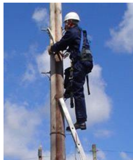
Figure 34 - shows right leg on lowest step and about to move onto pole & swing left leg onto next step.
