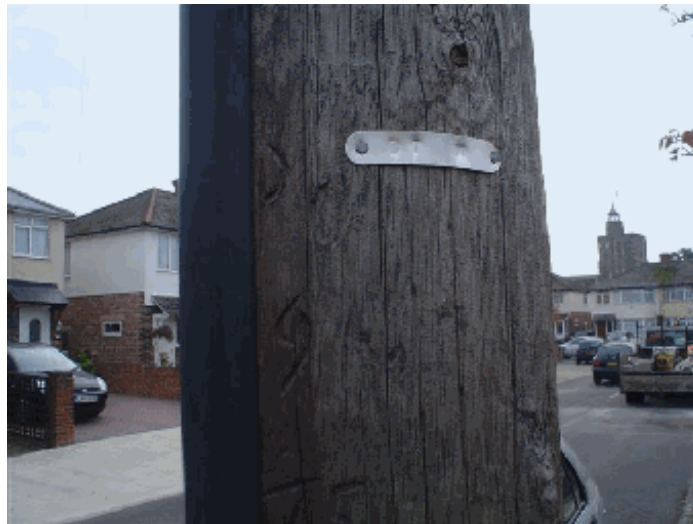
Figure 4- Aluminium strip fitted to same pole at the 3m point
