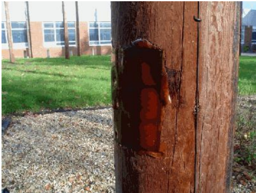
Figure 36: Resin repaired area
