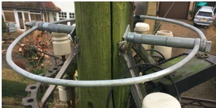
Figure 12 – Halo Ring fitted
