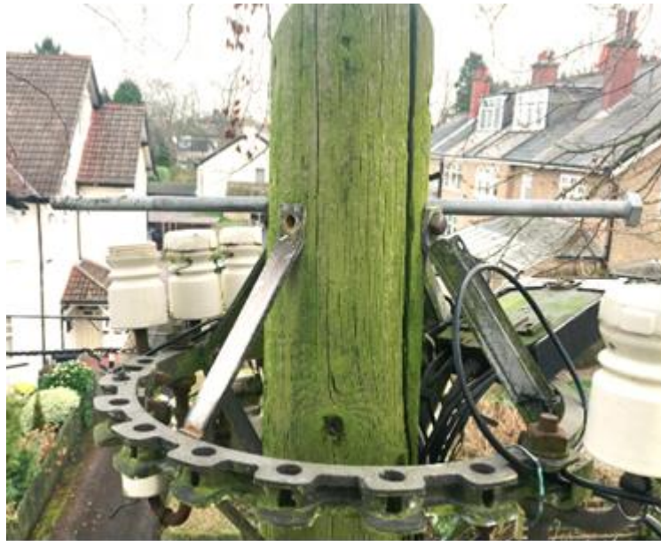
Figure 11 – Bolt sleeved through pole
