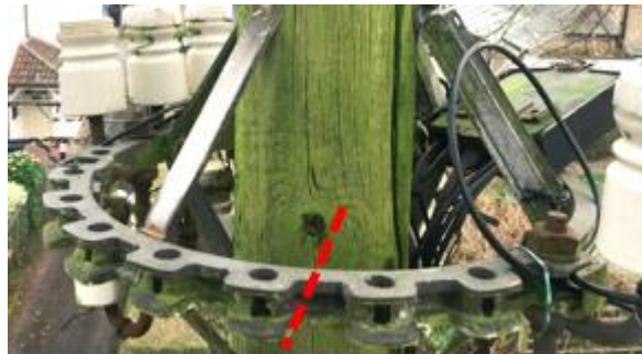
Figure 15 – Saw cut line
