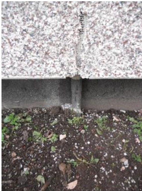
Figure 8 – EWI clad over Gas Feed
