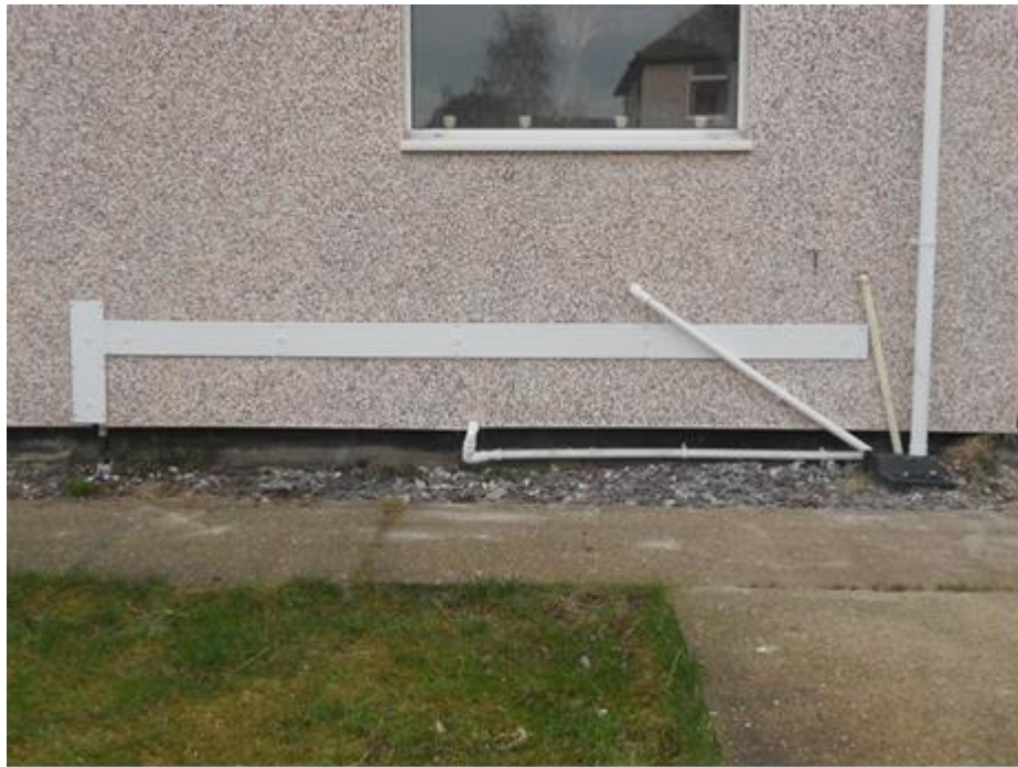
Figure 7: Gas feed in vented conduit
