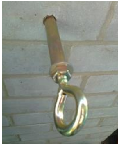
Figure 4 – Eyebolt 2C in advance of EWI
