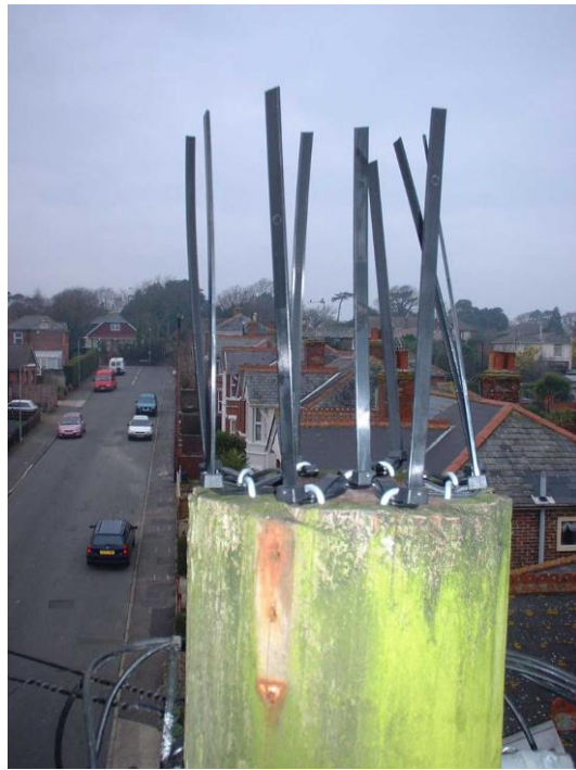
Figure 2: – Showing straps used as a bird deterrent
