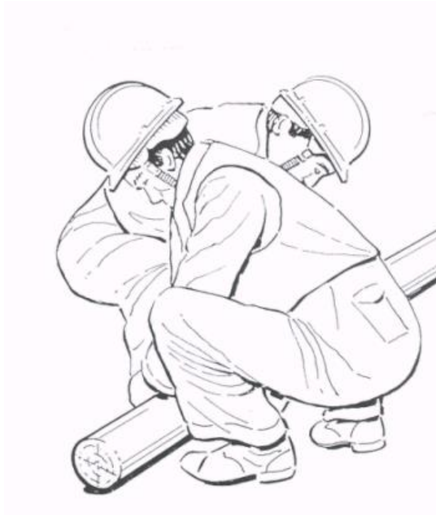
Figure 8: Preparing to Lift Pole Tip
