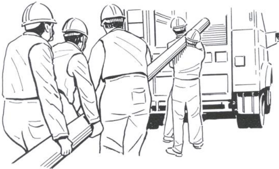
Figure 12: Loading Pole onto Vehicle (1)
