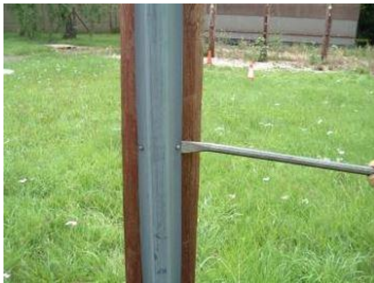
Levering the nail using a Wrecking Bar
