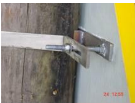
Bracket mounting on back of pole
