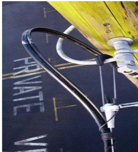
Figure 61 Attachment to Ring using Telenco BWC 25
