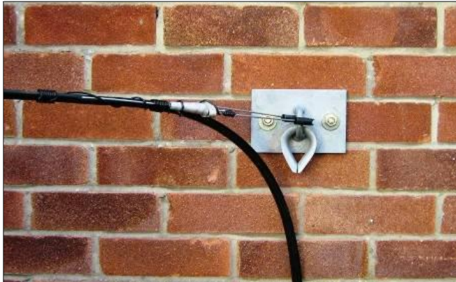
Figure 3 - Positioning a Plate Wall 5A on brickwork using Bolt Expanding 2A
