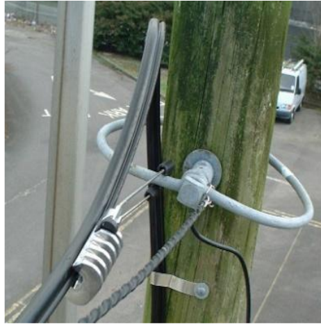
Figure 60 Attachment to Ring using Telenco AC7-200
