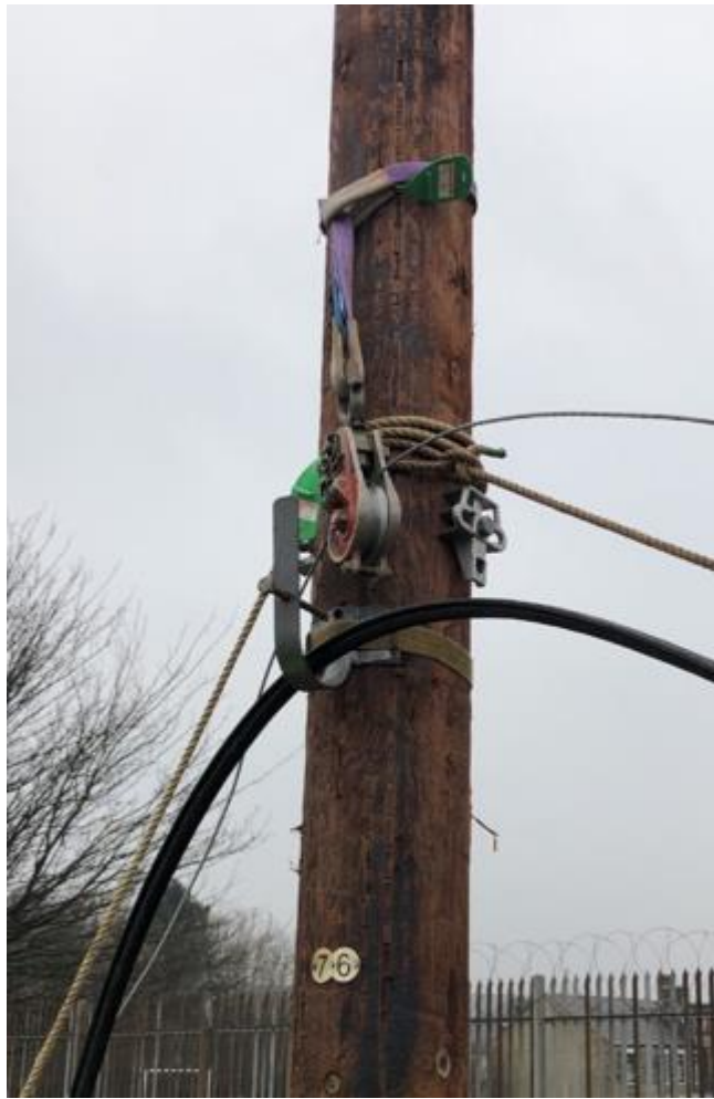
Figure 100 - Pole Top set up with a temporary back stay
