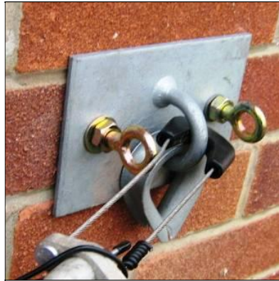
Figure 4 - Bail wires fouling the eyebolt
