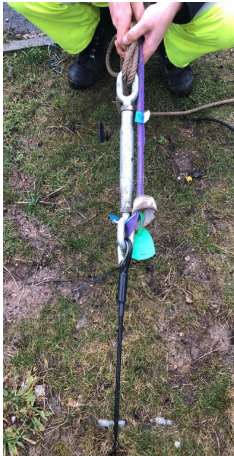
Figure 98 - Set up of a temporary back stay using the Anchor Stay 2 (Platipus)
